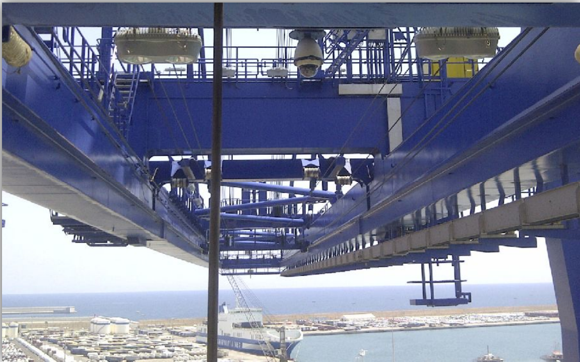
View of some 400WP on one STS at 52m height. TCV. Valencia. Spain
