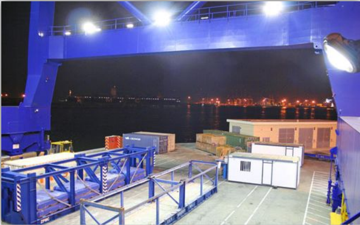
View of lighting level achieved under Girder of a STS Superpanamax. 300lx with 65% energy savings. By EDAE engineering, at TCV Terminal. Valencia. Spain
